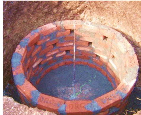
Upper layers in single brick with honeycombing in alternate layers
