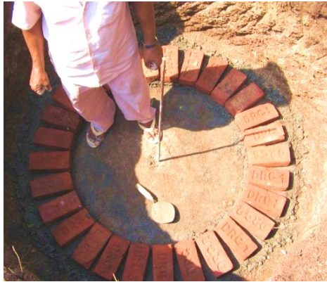
The first layer in 9" Brickwork
