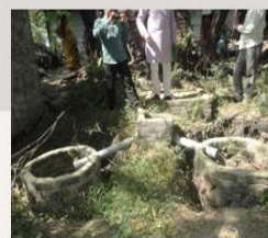
Pits smaller than required
