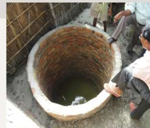
Pits smaller than required
