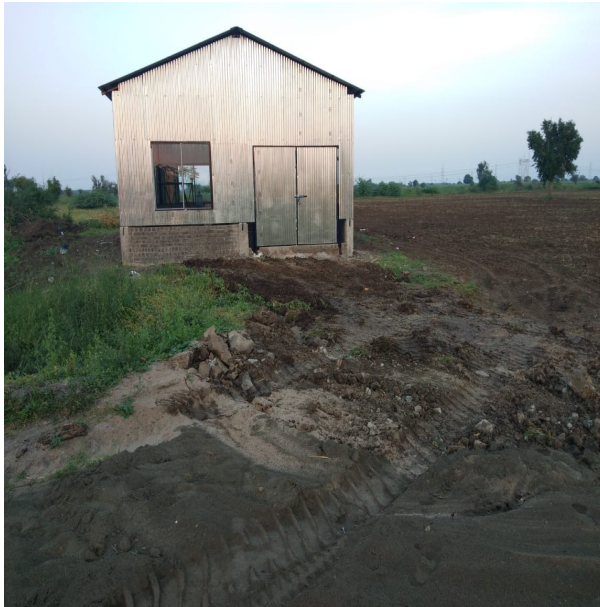
Model shed for dry waste
